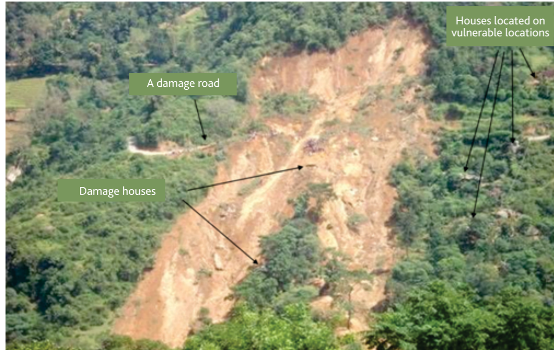
Fig 5.2: Human intervention into vulnerable hill slopes and landslide disaster in Sri Lanka; Kiriwanaella, Walapane landslide in which 12 people were killed and 5 houses were buried - Jan. 2007;
